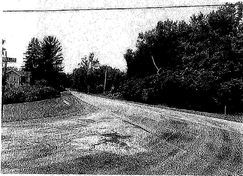
North Bergen Road at Merrill Road, looking West.
