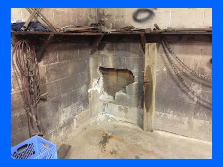
Wall opening to allow for plow to fit in the south bay
